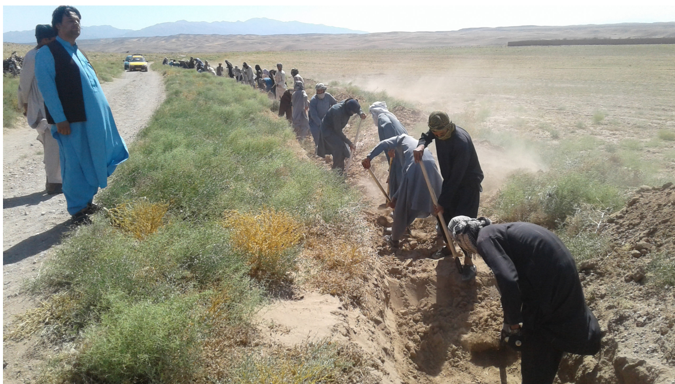
Water Canal rehabilitation in Injil district, Herat province
